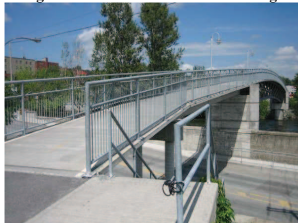
Figura 2 - The Sherbrooke Footbridge
