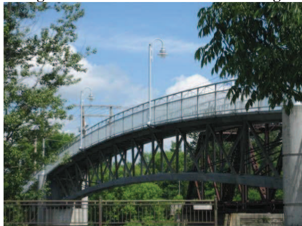
Figura 1 - The Sherbrooke Footbridge
